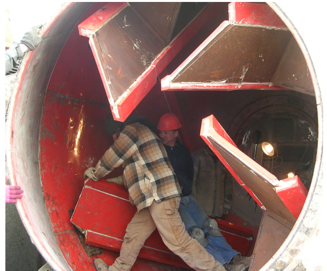
Durex wrap-around blade liners are installed on a Con-E-Co drum mixer
